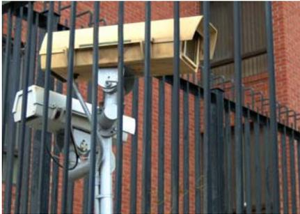
Movable cameras while very useful in the right situation can also be useless and even harmful to the overall security of your property if used in the wrong situation or environment. PTZ's are most efficient when used to supplement an already well designed surveillance system. For example, if you rely solely on the PTZ for coverage you may be disappointed when your camera is facing the wrong direction when you need it most. However if you have designed a
